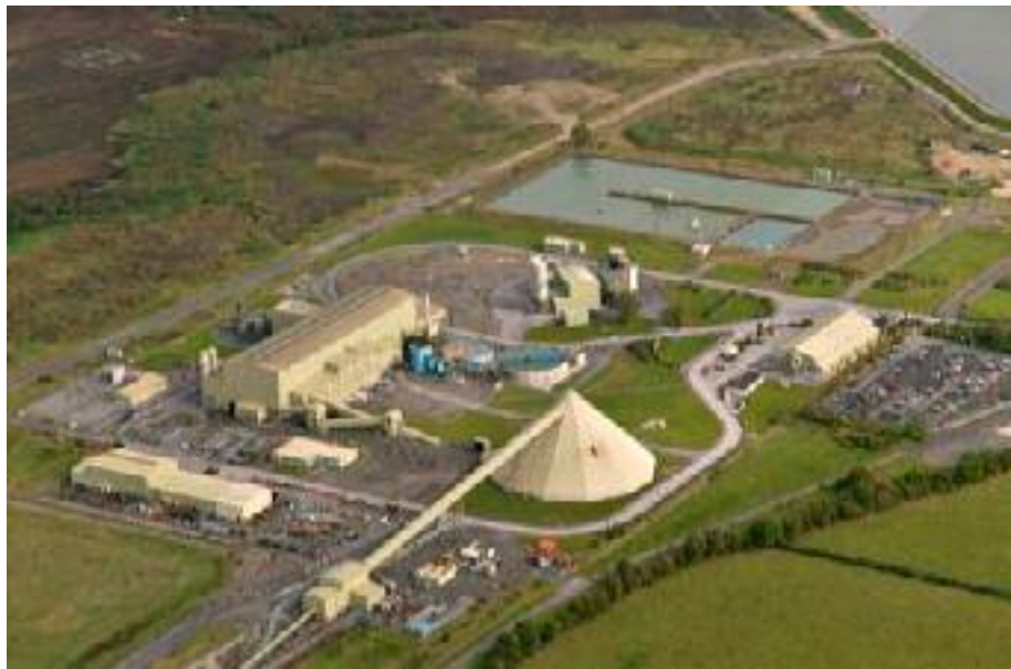
Fig. 1 - The Lisheen Mine at Moyne, Co. Tipperary
